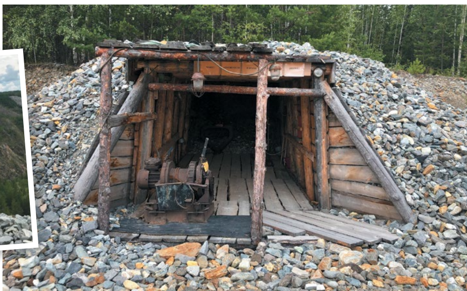
4: An old mine entrance that is no longer in use stands as a testament to how the forest reclaims the landscape with time.
