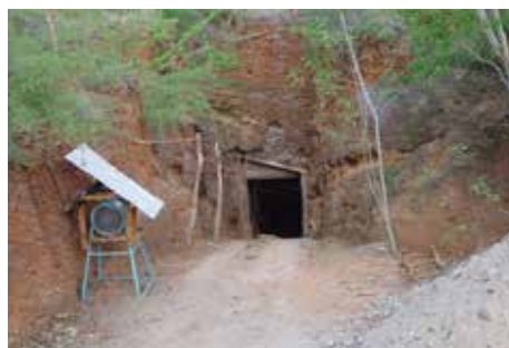
Entrance to No. 2 Tunnel.
