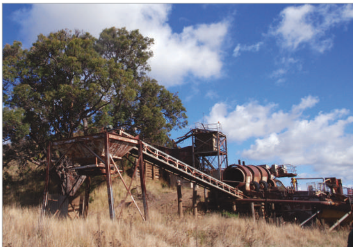
The sapphire processing plant at Reddestone Creek.
