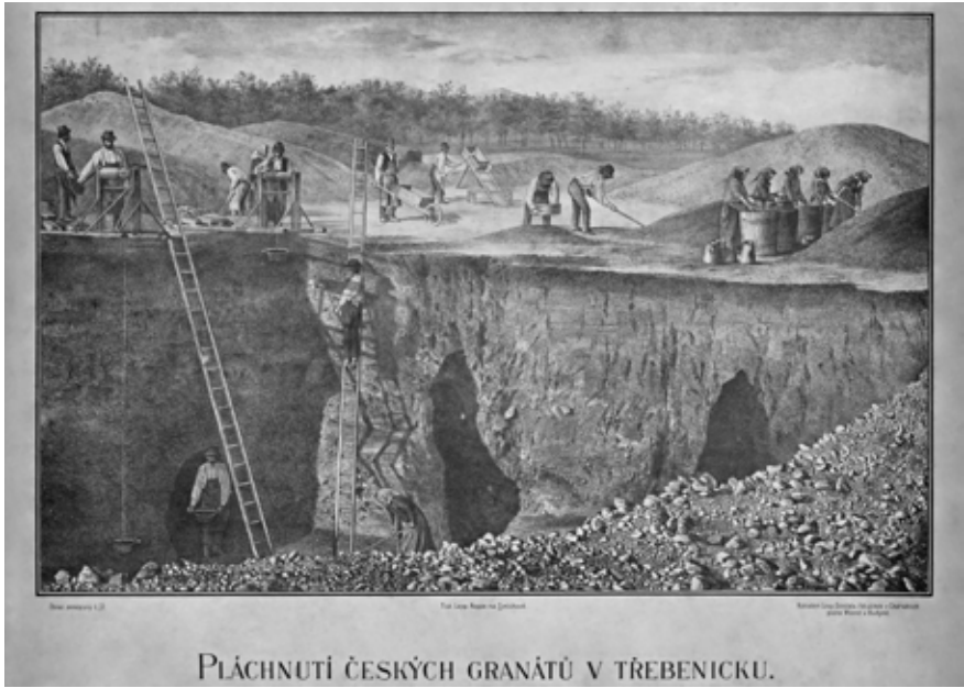
Figure 3: Mining of Bohemian garnets in Třebenice (Bohemian Central Highlands) around the end of the nineteenth and beginning of the twentieth century was done via both open-pit and underground methods. Image from the collection of R. Hanus.
